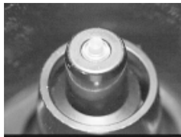
PB Fill connector before applying liquid leak detector.
